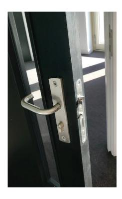
Mechanical opening by cylinder is always possible too, and the EL560 and EL460 locks are also compliant with EN179 and EN1125 Fire and Escape standards.
